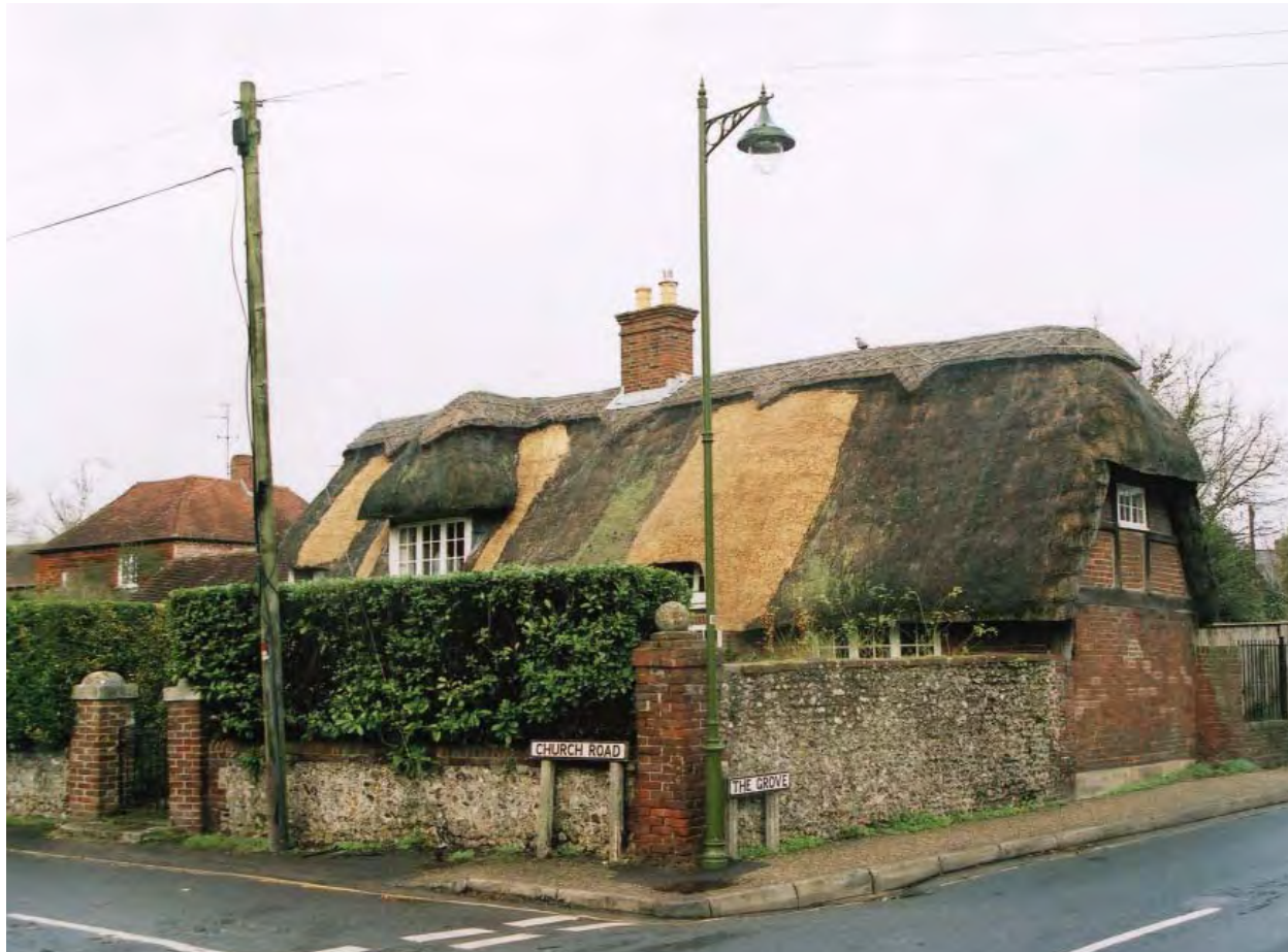
Overhead cables in Church Road
